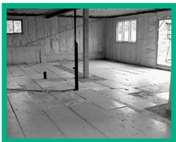
This underslab insulation made from scrap insulated steel door window cutouts scored highest in the CMHC test.
