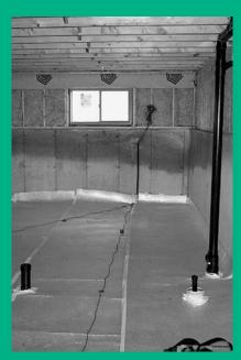
Bubble-pak insulation scored a rating of just over R-2.
