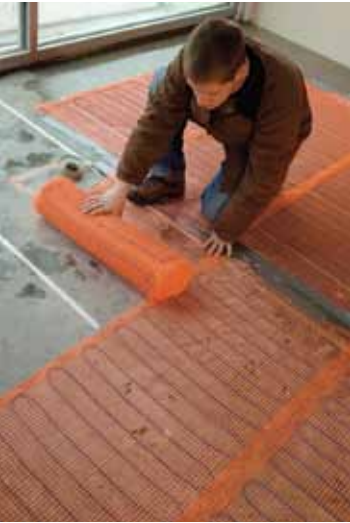
Roll out mat and secure to the floor.
