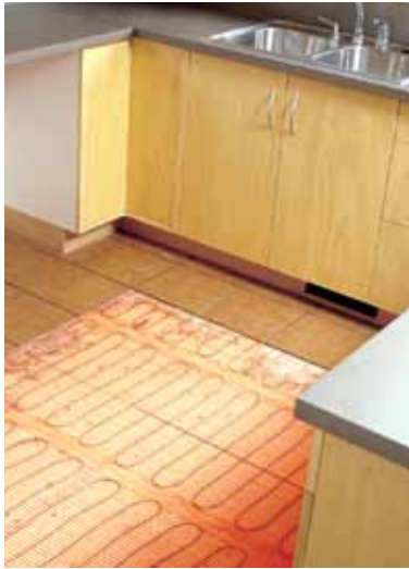
Trowel thin-set and lay tile.
